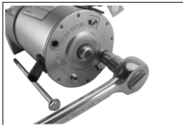
Figure 8-16. Removing Thru Bolts.
